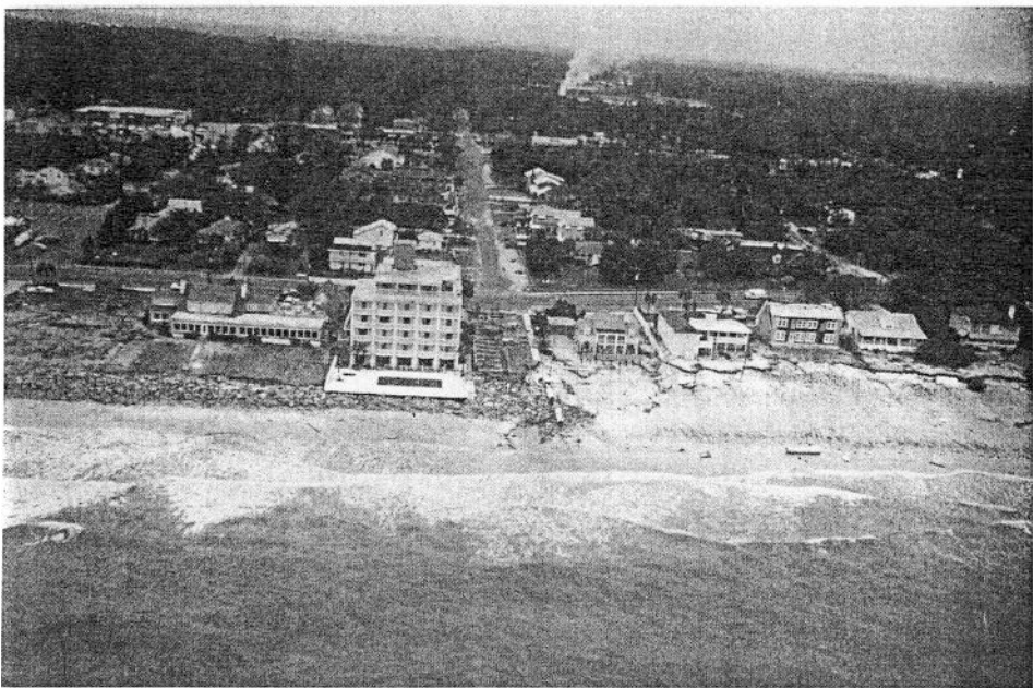
Fig. 8.2 South Myrtle Beach, South Carolina, after the passage of Hurricane Hugo in 1989. The buildings to the left, behind the rock seawall, were partially protected from the storm, but the beach is gone. To the right, the beach retreated, the buildings were flooded by the storm surge, but the beach is wide and healthy. This scene illustrates why society must ultimately choose between beaches and buildings.
